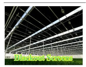
helps trap heat, while the aluminum strips reflect unwanted light back out of the greenhouse. These screens give very high energy savings of up to 70%.
