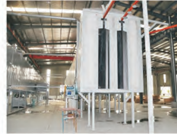
Tunnel curing oven and dry off oven
