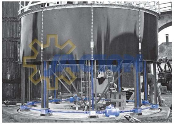
Each screw jack which support 2.5 ton load panels, travel stroke 1500mm, 20pcs worm gear screw jacks, low lifting speed, silo storage bolted tank application, outdoor ambient.
