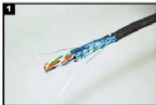
1 Strip back cable jacket using Linkbasic tool (P/N: TLD01) or equivalent.
