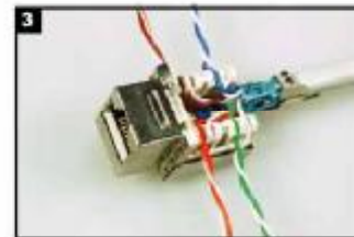
3 Insert each wire into the appropriate channel according to the color code on the module.
