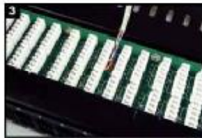
3 Check and ensure each wire in correct slot.
