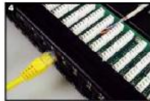
4 Insert the jack into the correct mounting location properly.
