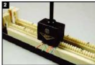
2 Terminate wires using Linkbasic tool (P/N: TLB01) or equivalent.
