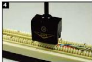
4 Install connecting block in the wiring block tightly.
