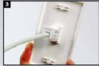
Align the jack to the slot.
