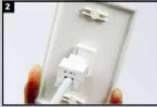
Carefully seat the jacks over the back of the faceplate.
