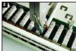
2 Terminate wires using Linkbasic tool (P/N: TLA01) or equivalent.
