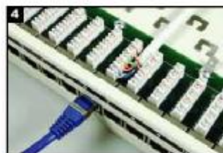
4 Insert the jack into the correct mounting location properly.
