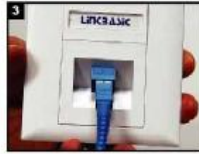
Snap the patch cord in slot.
