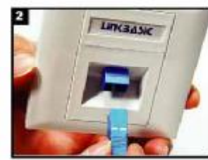
Carefully seat the adapter over the front of the faceplate.
