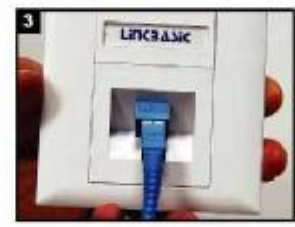
Snap the patch cord in slot.
